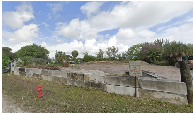
Figure 4. Existing Conditions (view from Nokomis Ave.)
