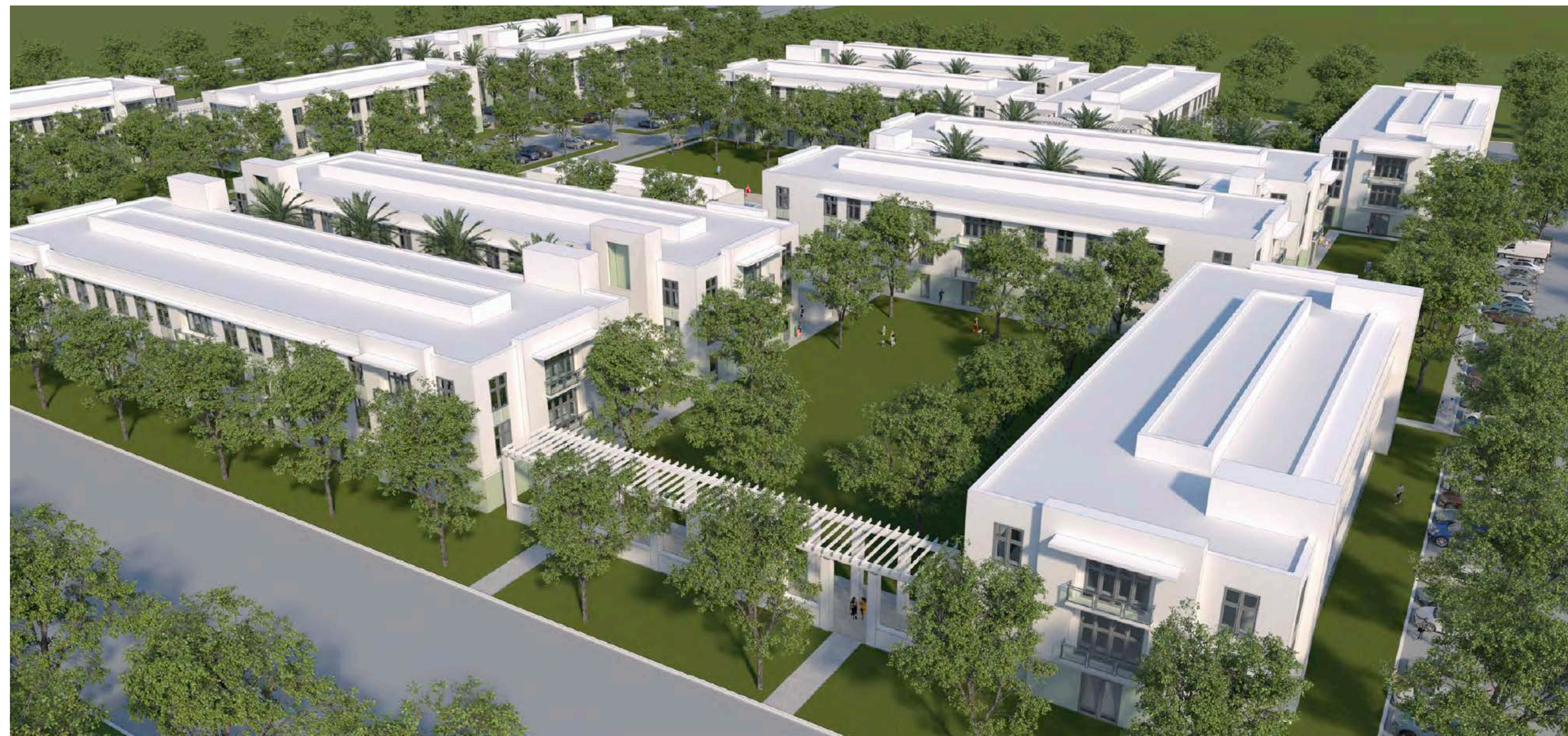
Westgate Gardens, Phase 1: Aerial Looking Southeast
