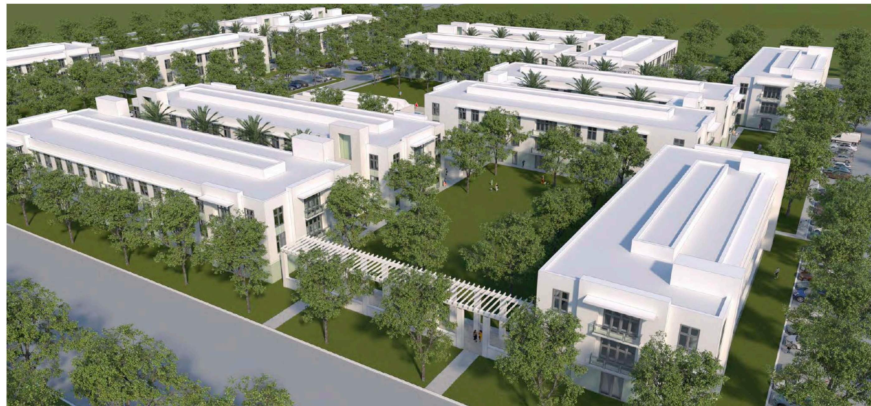
Westgate Gardens, Phase 1: Aerial Looking Southeast
