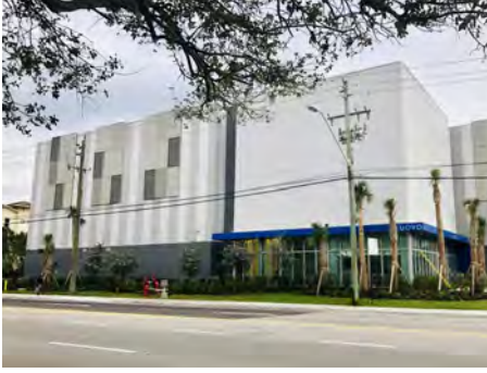
Uovo Art (Westgate Avenue) 2-story, 49,760 sf limited access art and antiques self-service storage
