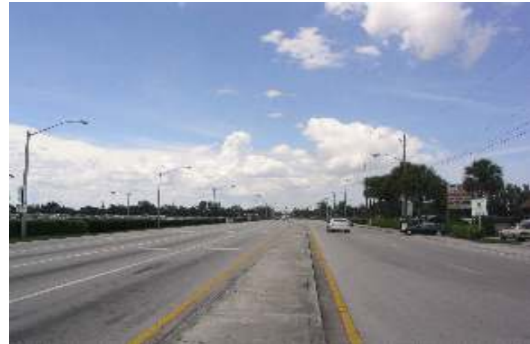
Fig. 2.11 Congress Avenue looking North
