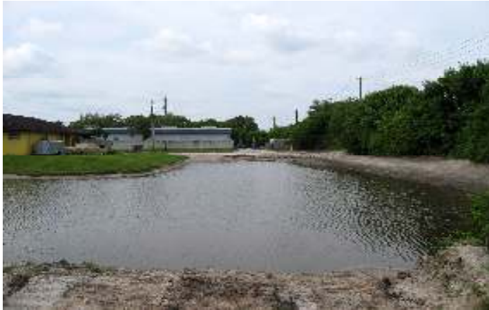
Fig. 2.8 Required Detention Pond on Chickamagua Avenue
